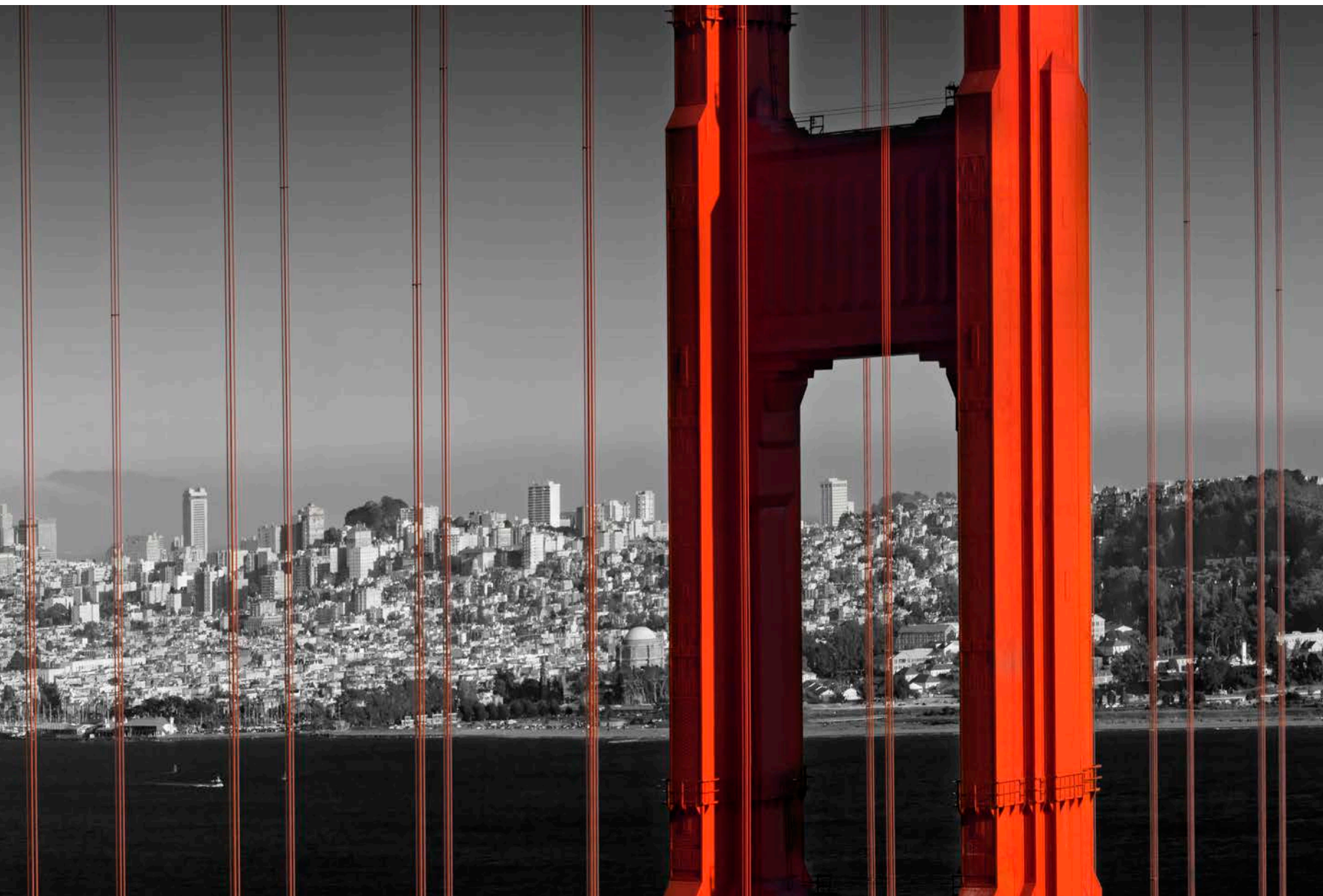
Golden Gate Bridge | Panorama
